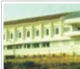
Verna, Goa for packaged pre-engineered water treatment plants and membranes.
